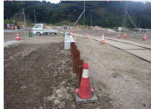
② 樋管本体内可撓鋼矢板①
