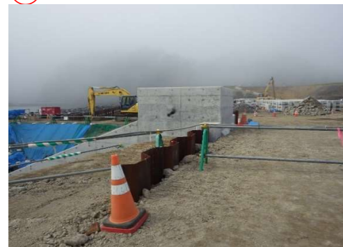
③ 樋管本体内可撓鋼矢板②
